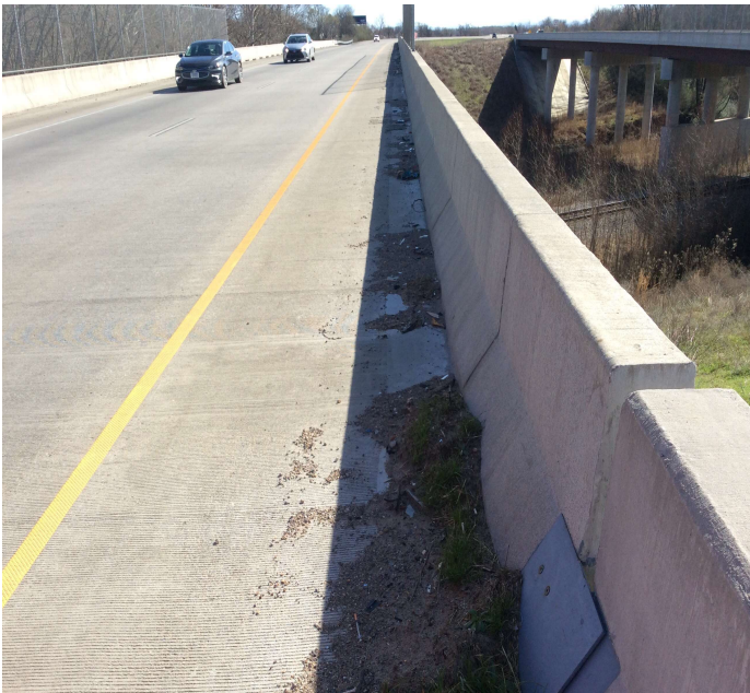
PHOTO 1 Description Gutters with debris accumulation.
